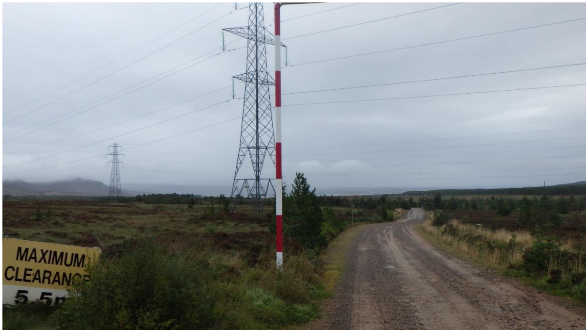
Photo 5: Shows the overhead lines crossing the access track (with a maximum clearance of 5.5 m) and view looking east
